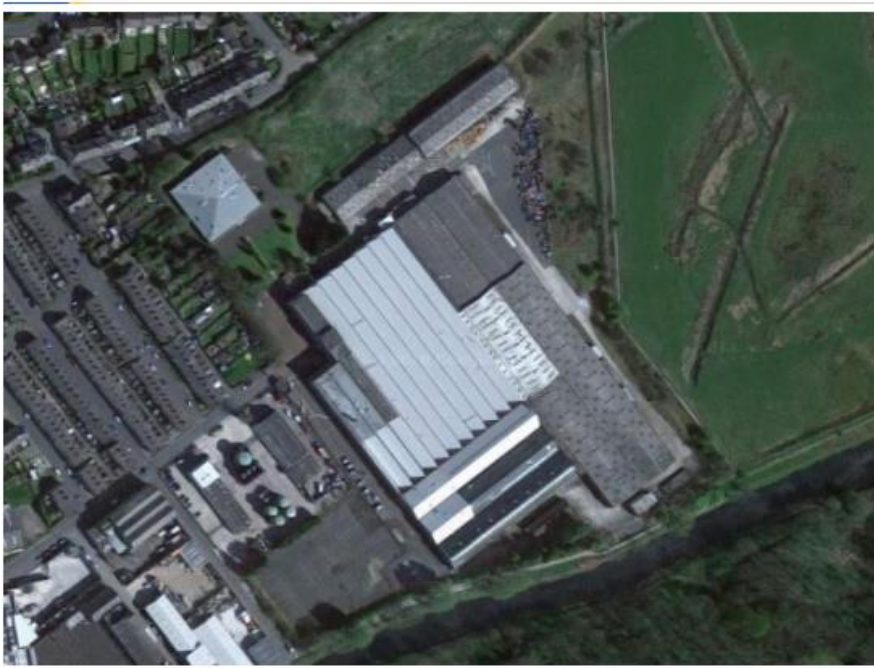
Homes England has already started demolition work on the former factory in Padiham
