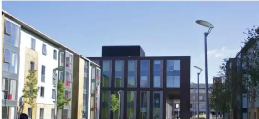
Major infrastructure plans to support new homes in Lancaster and the development of Lancaster University, including the new Health Innovation Campus, have received approval to be taken to the next stage.
